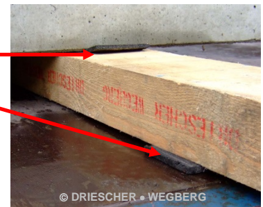
Betonfundament Concrete foundation
