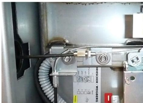
If installation of the metering cubicle is on the left side from the switchgear cubicle guide the Bowden wire from the left side into the straight end cover in the switchgear cubicle as shown on the picture left.
