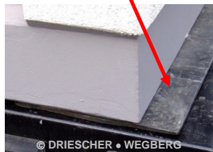
Betonstation Concrete station
