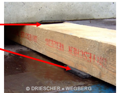
Betonfundament Concrete foundation
