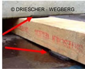
Avoid a displacement of the substation during transport with anti-slipping-mats. These must be put below the bearing points of the sub-station. In case timbers or pallets are utilized for the loading these also have to be placed onto anti-slipping-mats.
